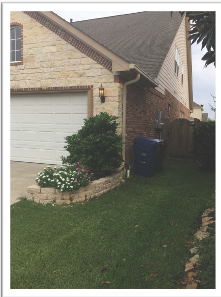
Storage Location Violation (In View - Side of Home)
